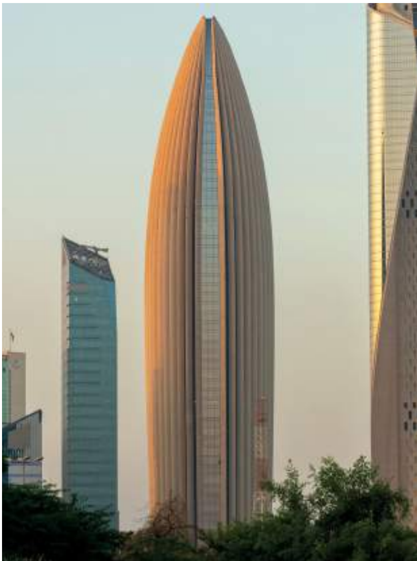
NATIONAL BANK OF KUWAIT TOWER , KUWAIT CITY, KUWAIT
