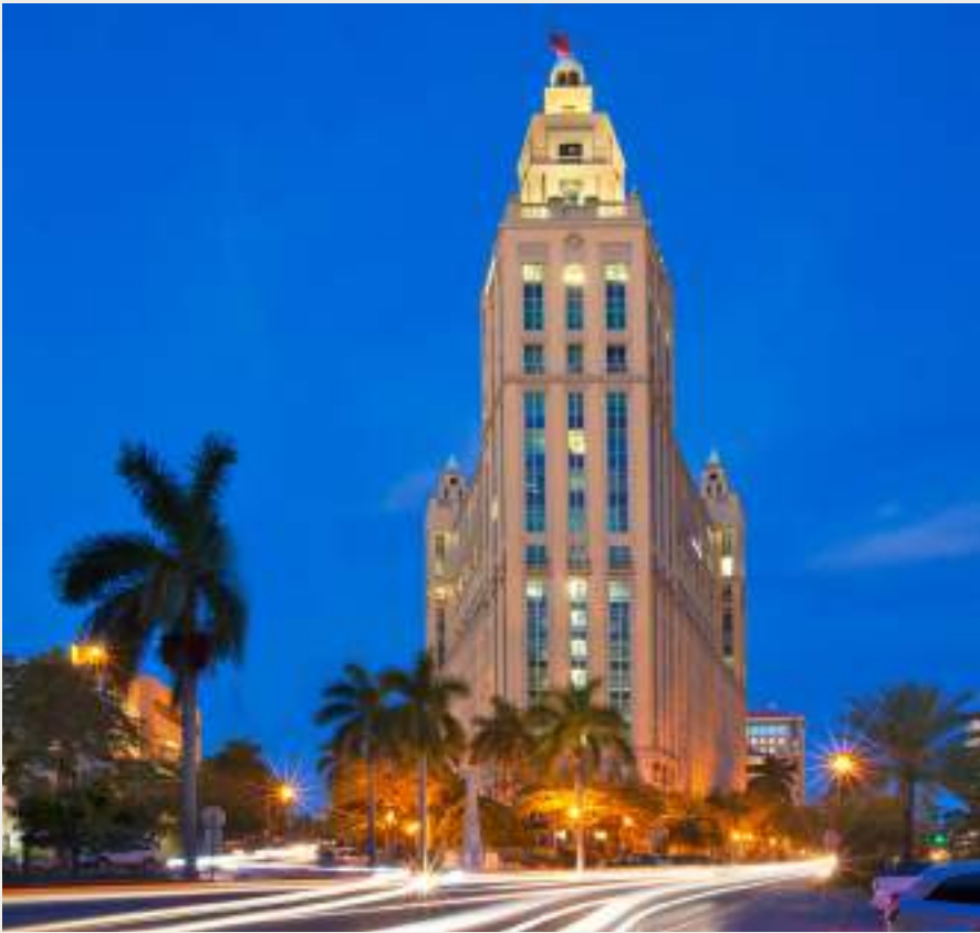
Alhambra Towers, Coral Gables, FL
